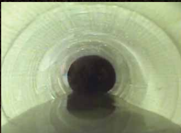
AFTER HAMMERHEAD POINT REPAIR
