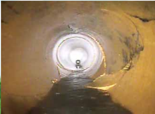
BEFORE HAMMERHEAD® POINT REPAIR
